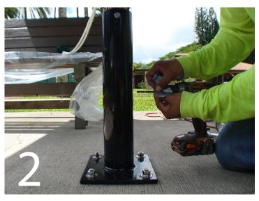
Using tape, mark your drill bit so that it is marked at half the width of what you are drilling through. At this point ensure that your umbrella is positioned correctly and use the tightening bolt to lock the umbrella in position. If you don't have a tightening bolt, use shims to wedge the umbrella pole in place and keep it from spinning.
