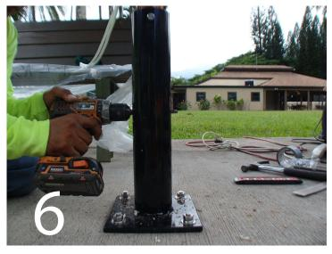
When you meet the other hole halfway, continue until your drill bit pops out the other side. Continue to drill out the hole until the drill bit slides in and out smoothly.
