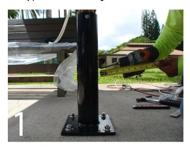
Measure the width of whatever your through bolt is going through. You will take this measurement and divide it in half. This is the measurement you will mark on your 5/16" drill bit. In this example, our through bolt is going through a 4" pipe, so we will mark our drill bit at 2". Your through bolt may go through something larger or smaller.
