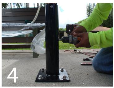
Drill until the tape reaches the outside of your base or table coupler. If you are drilling through the stainless pole of the umbrella, use cutting fluid to keep your bit from overheating and dulling quickly.
